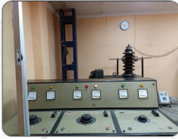
HIGH VOLTAGE-MILLI VOLT-TEMP. TEST ASSEMBLY
